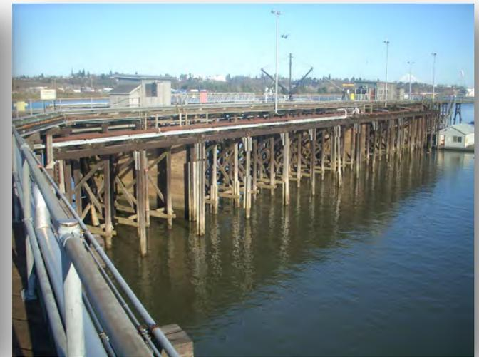
Olympic Pipeline built in the 1960s without seismic design standards
